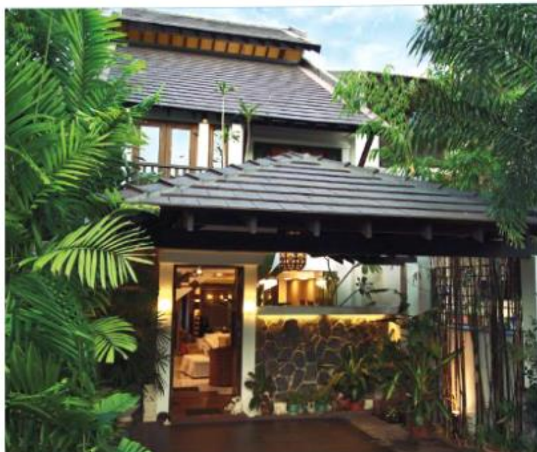
A double-storey inter-terrace transformed into a tropical villa
